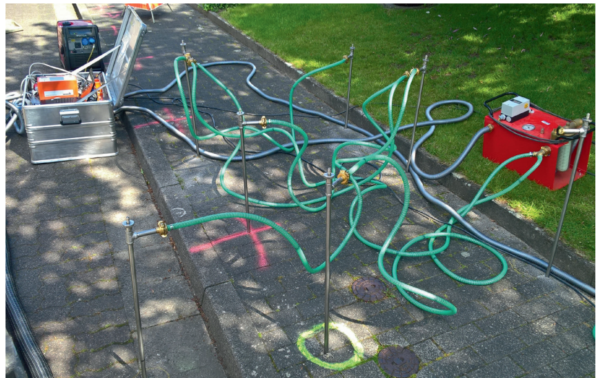
Figure 2: Measurement Using the Suction Method at a Buried Pipeline
